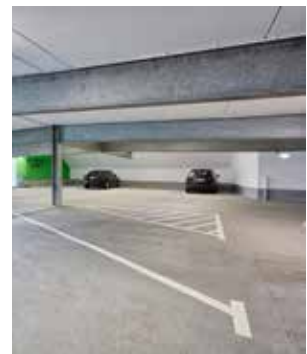
UNDERGROUND PARKING AREA
