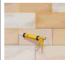
Natural stone joints
