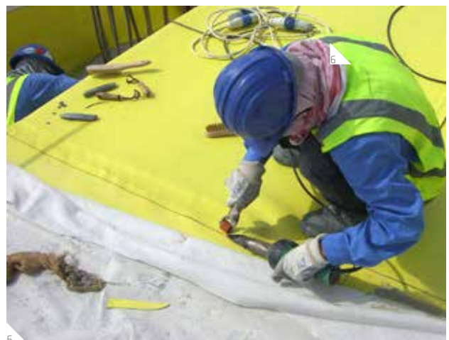
6 Compartmentalized sheet membrane systems
